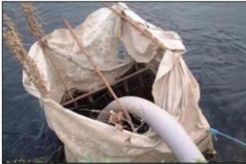
A screened abstraction point using terram fitted over a fabricated support frame.
