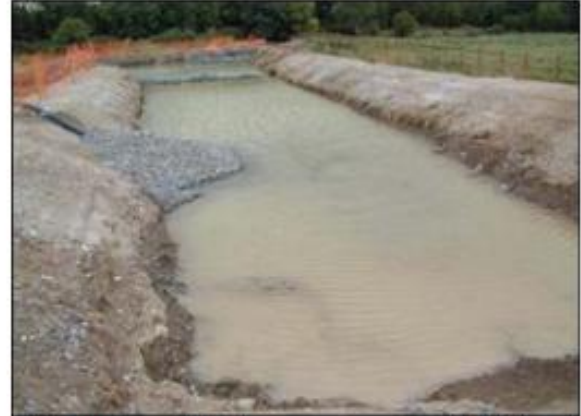
Silt control pond. Note hose conveying pumped silt laden waters with its outlet positioned within the gravel mound thus ensuring no disturbance of pond contents.
