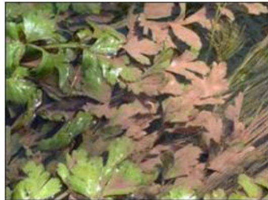
The practical impact of poor silt control.
