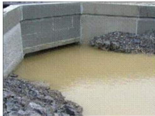
Is the culvert adequately sized?
